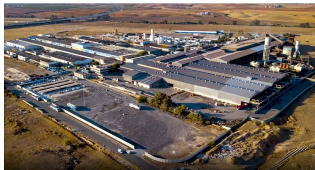
Figure 1: Situation prior to the works
